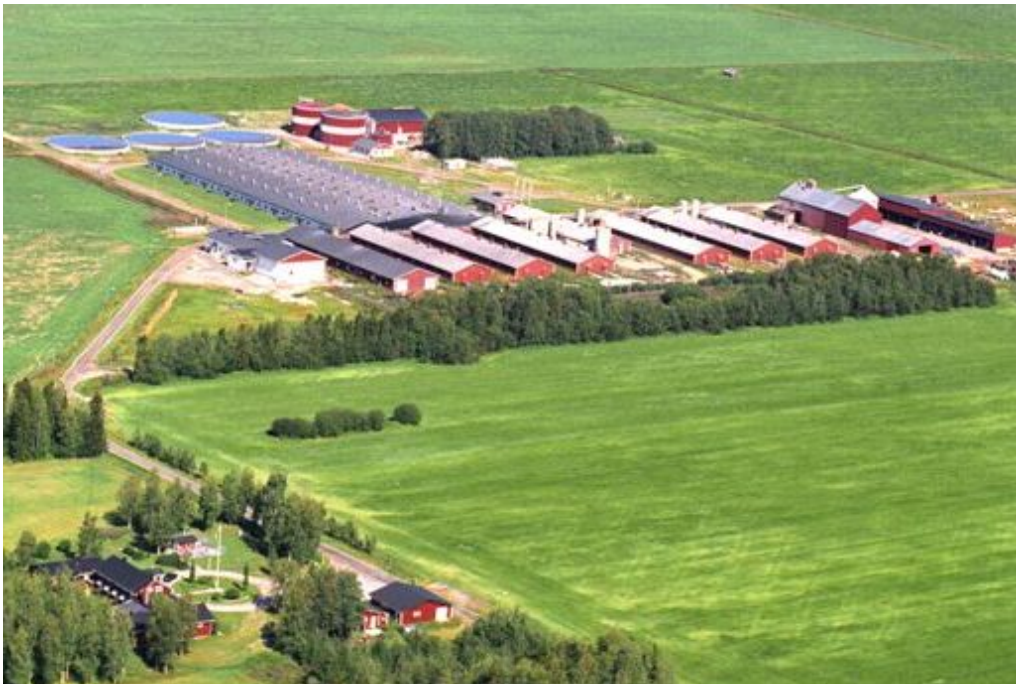
Figure 1 Photograph of the biogas plant in Alvik
