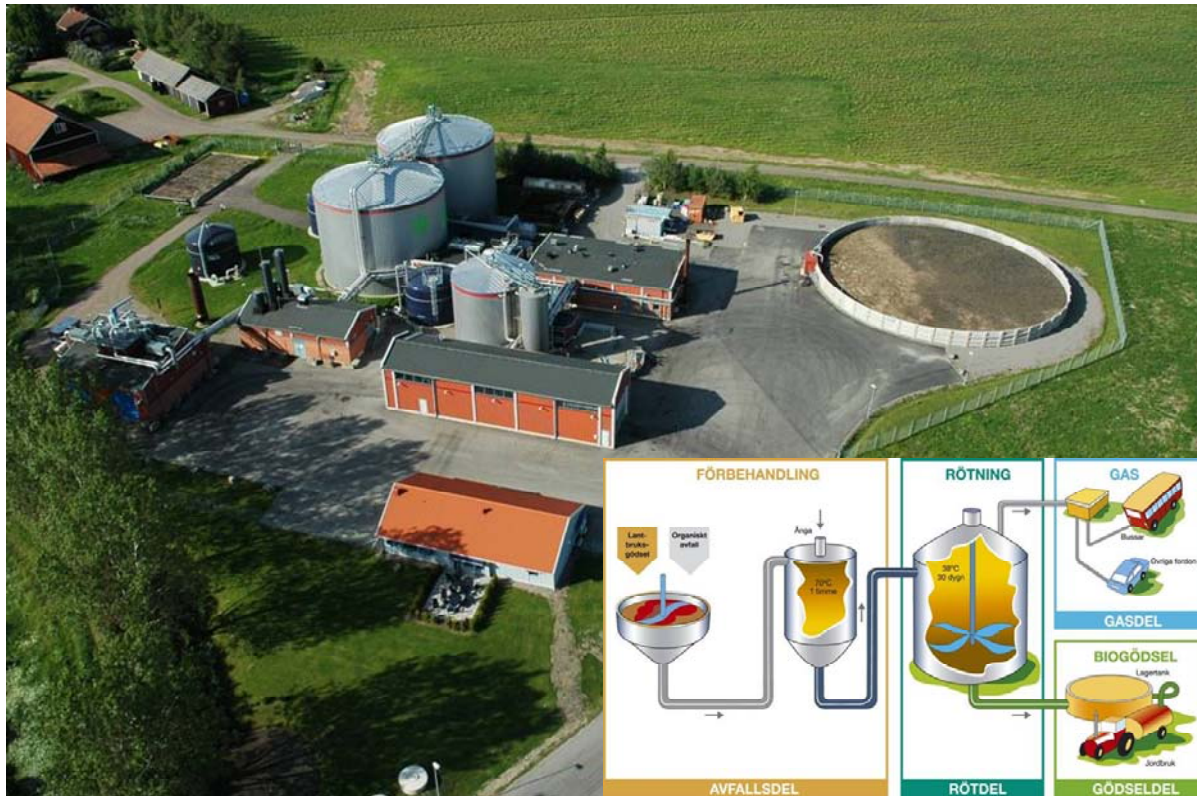
Figure 2 Aerial photograph of the biogas plant in Linköping, with a schematic diagram of the plant
