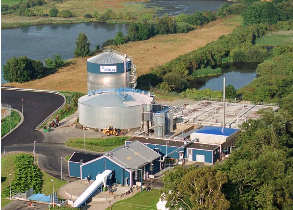
Figure 1 The biogas plant at Karpalund, Kristianstad
